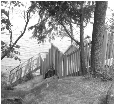
New Stairway at Anglers' Cove
